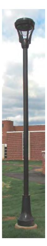
Replacement of any antiquated, inefficient pedestrian walkway lighting is recommended. Metal halide lamps in cut-off luminaires mounted to poles are recommended. Color/finish should be consistent campus wide. Avoid the use of bollards due to vulnerability to snow removal operations and vandalism. The two types illustrated here exist on campus and are recommended for campus wide installation as new projects or replacement opportunities arise.
