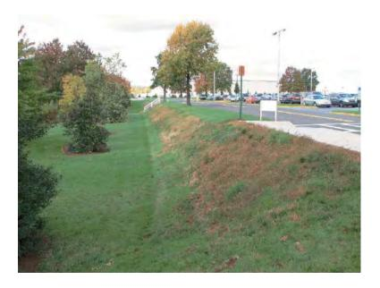
The degree of slope on existing bank makes maintenance of these areas difficult and hazardous. Recommend the replacement of grass with mulched planting beds.
