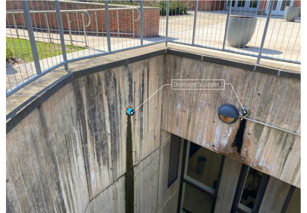
Looking down into the Sunken Courtyard foundation walls and drainage scuppers
