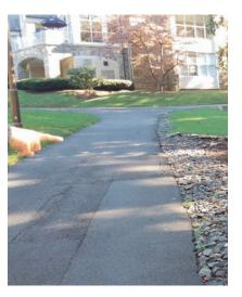
University standard for sidewalk surfacing is concrete. A strategy for replacing bituminous sidewalks should be developed and implemented.
