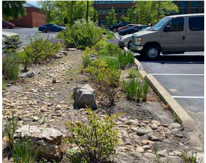
Stormwater Swale at the Stuckeman Family Building
