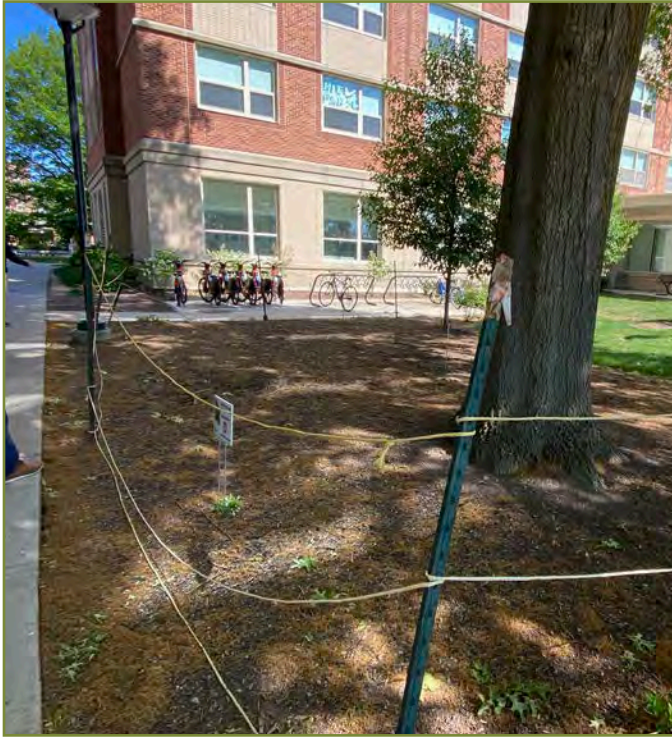
An example of tree and soil protection adjacent to an existing construction project.
